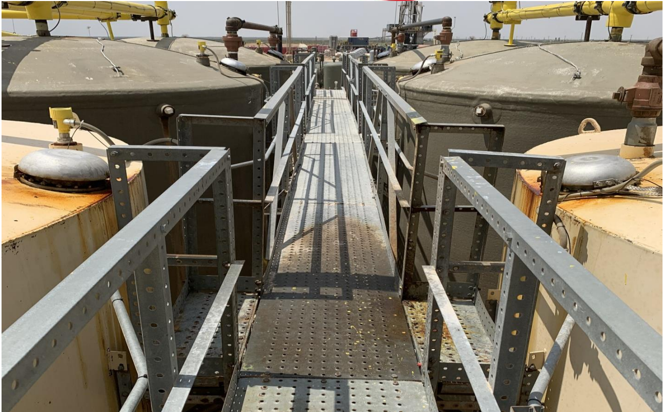
Tank battery catwalk to access hatches
