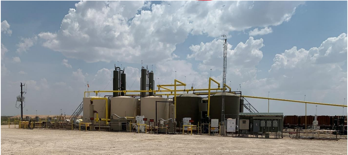
Test well site in West Texas
